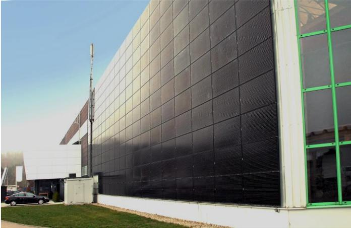
A component of the company's energy transition at Mayer: a combination of façade-integrated photovoltaic installation and the VARTA storage system.
