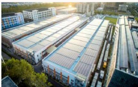
4MW Testing PV Plant
